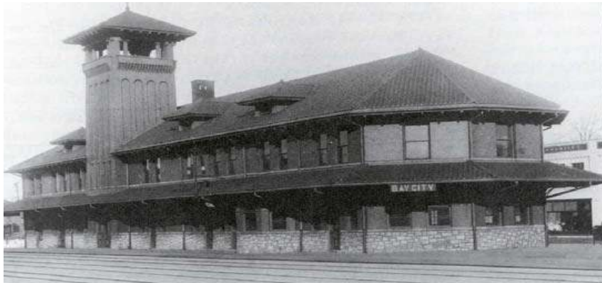
Historic undated photo, West elevation
